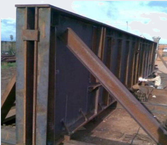
Boiler top support beam
