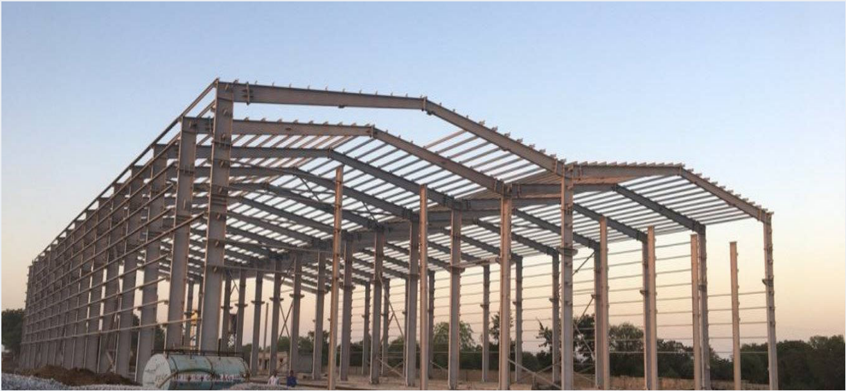
Body & Bogie repairing workshop , Project : Western Railways , Ratlam Division Size : 23.0 m x 100.0 m x 2 Spans , Weight : 750 MT approx.
