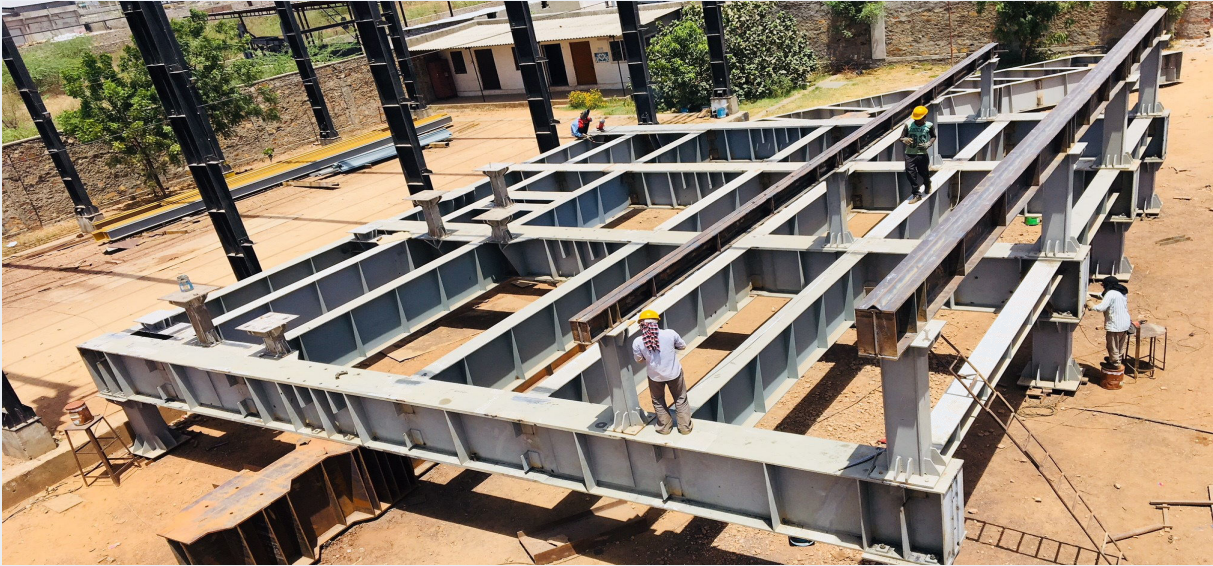
Base Frame for Boiler Module for Project : Dangote Oil Refinery Limited Size : 13.0 m x 45.0 m , Weight : 140.0 MT
